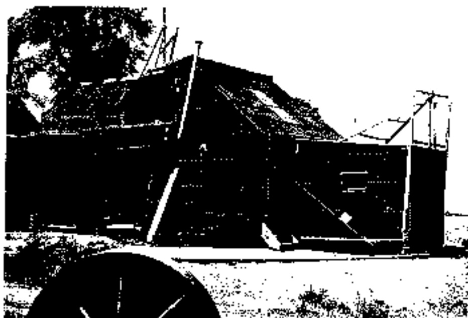
12.3 The hinged portion of the Black Maria's roof could either swing open for filming.
