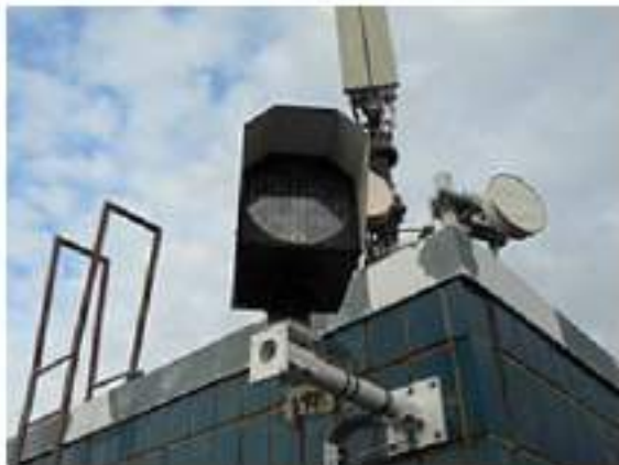
Laserlink point to point optical wireless network
