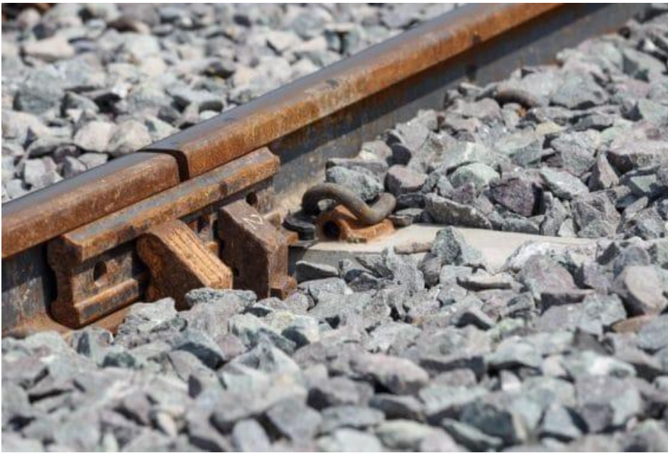
Fig 2: Basalt and Trap as Railway Ballast
