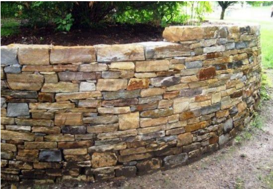
Fig 10: Quartzite Retaining Wall
